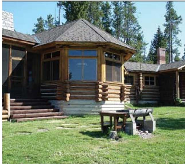
Berol Lodge at UW-NPS Research Center
